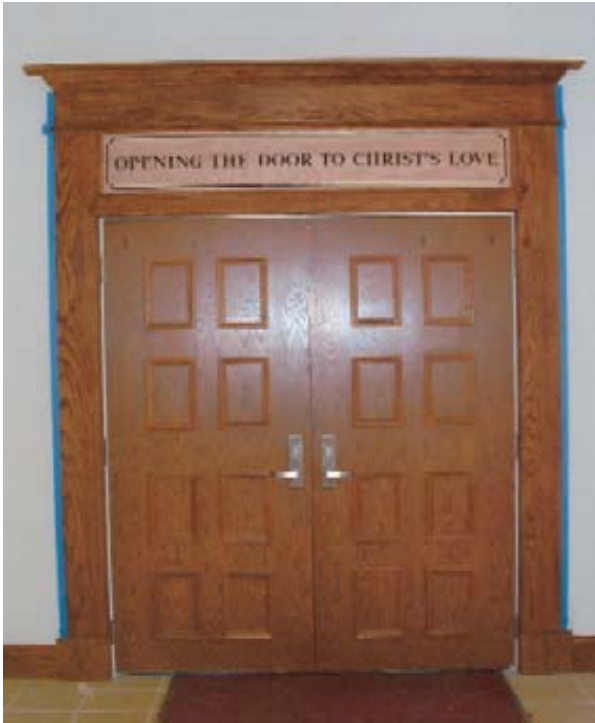
The new doors
