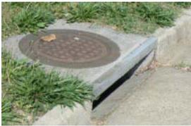
Storm drain inlets are located at low spots along the roads to prevent flooding by carrying rain and melting ice or snow away from our streets. This storm drainage system empties the water and all wastes collected by the water directly into our watersheds. **The storm water is not filtered at a treatment plant!**
