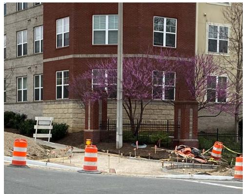
To slow traffic on the approaches of the new crosswalk, Memorial St. width will be visually narrowed using pavement markings and with the addition of a wide, raised pedestrian refuge island.
